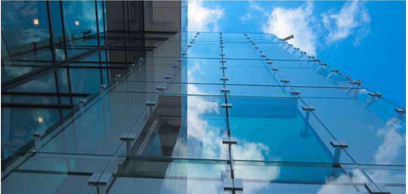
The 12 floor, 17.624 m 2 (189,700 sqft) building exploits the highly transparent characteristics of SentryGlas® to complement the low-iron glass used in the weather shield on all aspects of the building.
