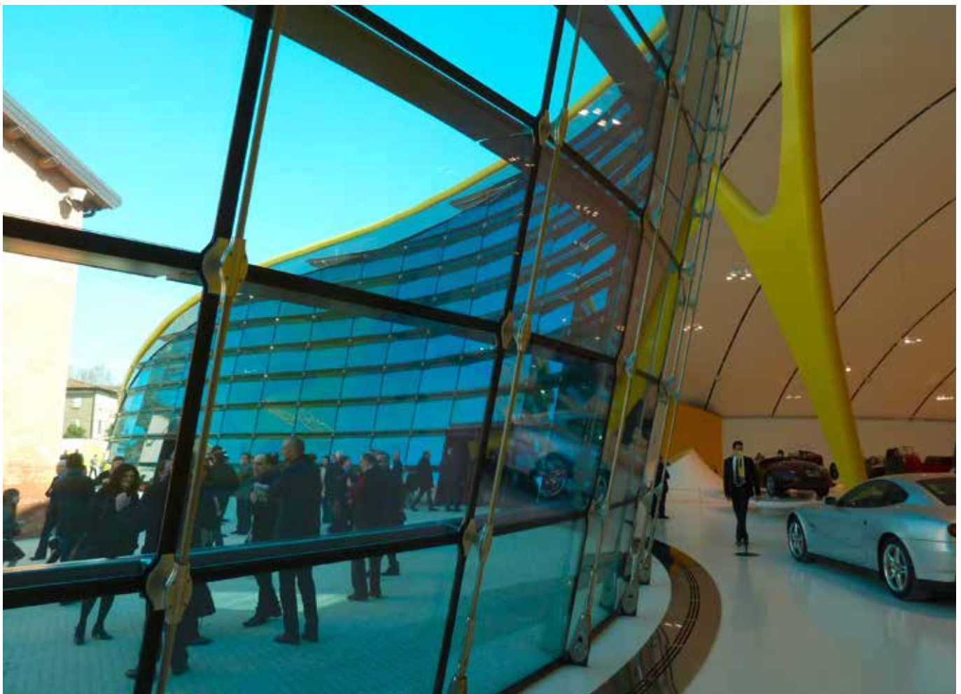
The opening of the Enzo Ferrari Museum. A set of 32 mm (1¼") vertical stainless steel cables supports the flat insulated glass panels. Glass make-up comprises a 10 mm (3/8") fully tempered glass pane on the outside, with two 6 mm (¼") heat strengthened glass panes laminated with 1.52 mm (60 mil) SentryGlas® interlayer on the inside.
